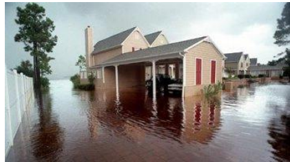
Residents of Garnier's Cay on Shalimar Drive ended up with more waterfront property than usual after heavy rains and waves pushed Garnier's Bayou into their yards.
